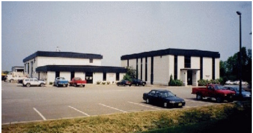
SCMUA Administrative and Maintenance Complex
